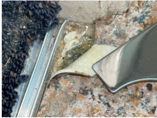
View of layers under multicolor vinyl sheet flooring
